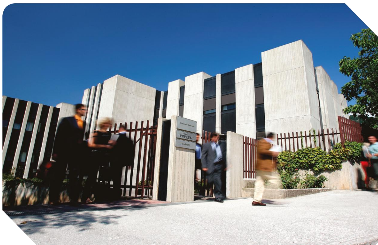
Figure 1 – Headquarters of Colacem S.p.A. - Gubbio (PG)
